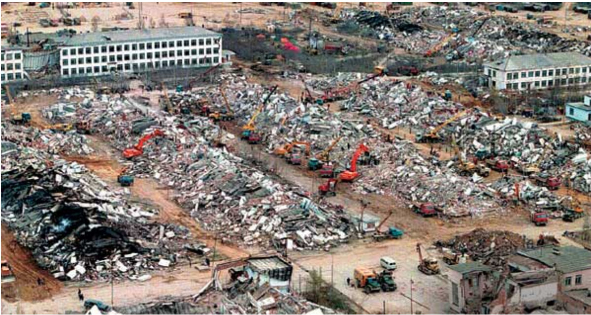
Fig. 8. Heavy damages by the Neftegorsk earthquake
