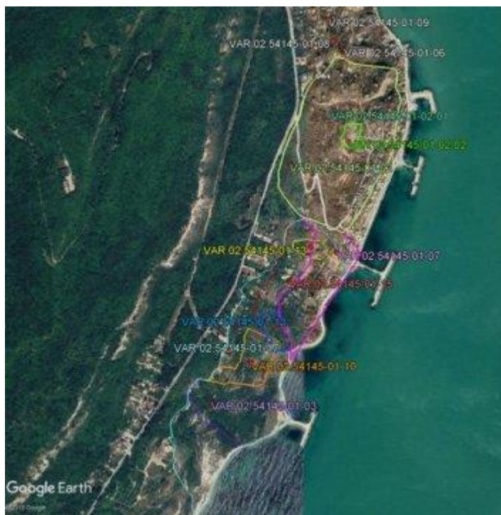
Fig. 6. ID codes from MRDPW register and the boundaries of the investigated landslides in the area of "Fara" landslide
