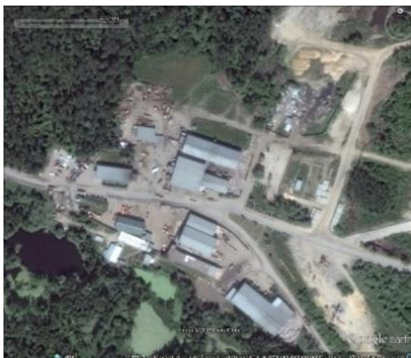
Fig. 4. The image of the landfill
